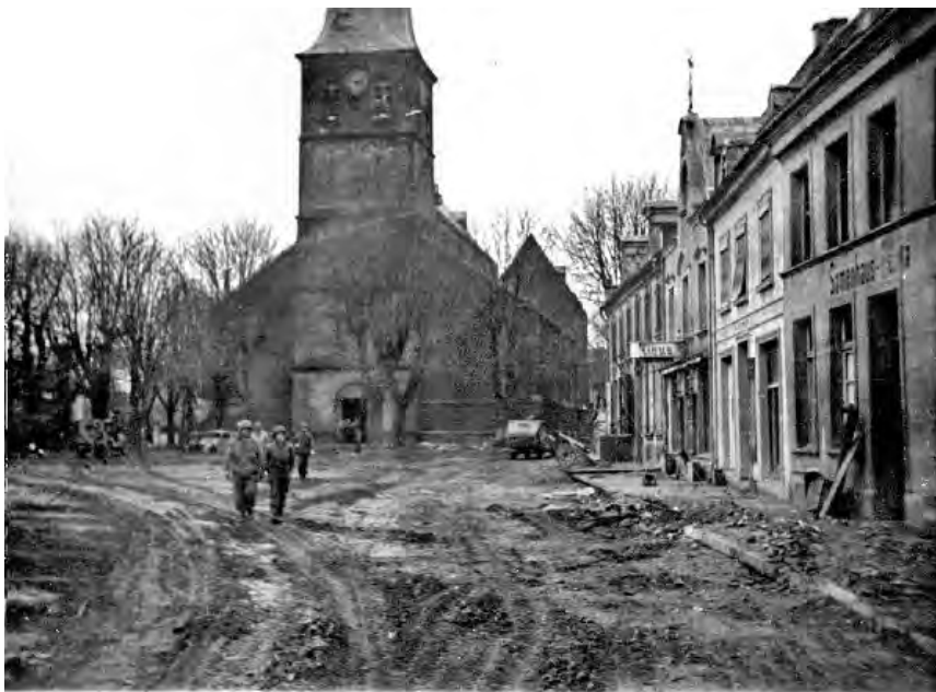
14. Church and square in Rheinberg around which Capt. Kelly rode in his tank in the first penetration of the town.
